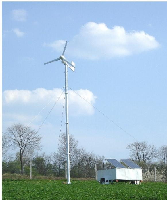
**Figure (1):** Mobile hybrid power supply (1 kW installed power)
